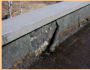
Deteriorating waterproof roof (leakage)
