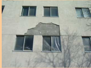
Masonry chipping on outside walls
