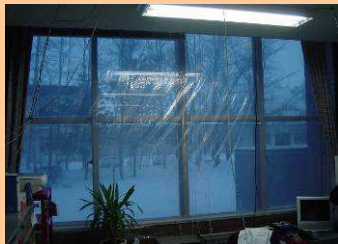
Iron sashes allow drafts (reinforced with vinyl)
