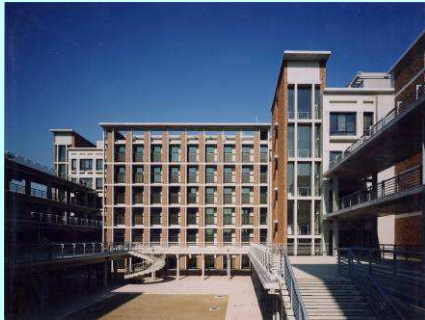
General research building
