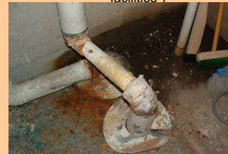
Rusty pipes, damage to lagging material
