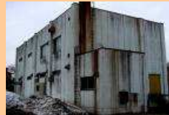
Ageing facilities (exterior)
