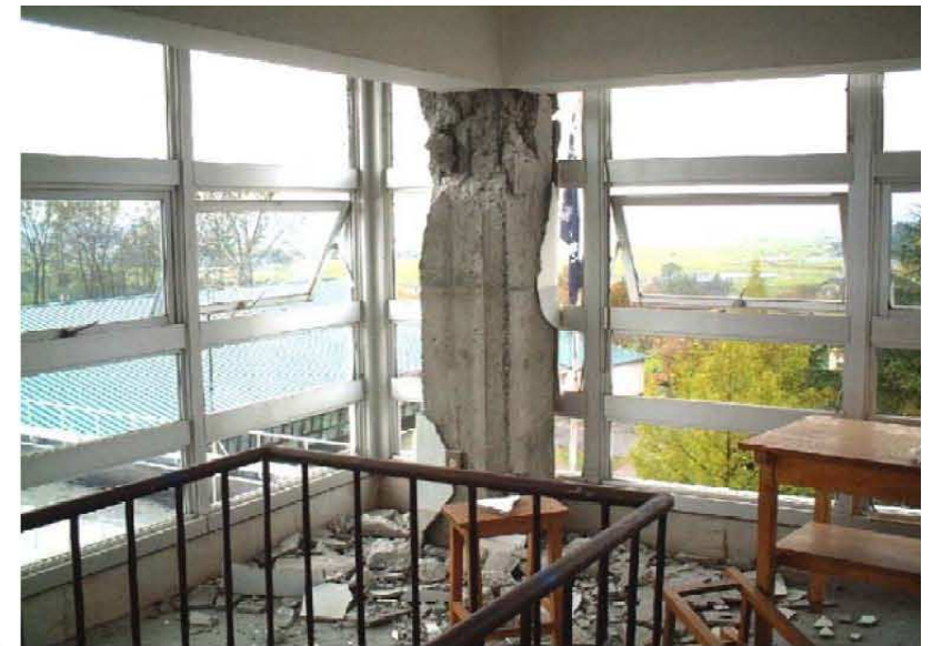
Facility damaged by earthquake
